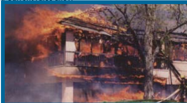
Office Building Fire in Pennsylvania- Electrical Fire Above Ceiling of 2nd Floor- Full Collapse of Roof Within Minutes - $4,000,000 Loss (Reprinted from NFPA Journal)
