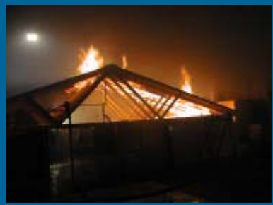
Task Group Fire-Test in 4/12 Roof Slope- This was considered acceptable
